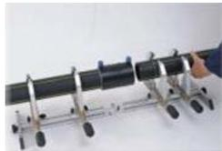
Using pipe clamps, secure the fitting and pipes in place to prevent movement of the joint during the fusion and cooling cycle. Ensure that the pipes and fitting are properly aligned (with no angle between pipe axes), are not subjected to a bending stress, and are not left to support their own weight in the fitting or weight of the fitting.
